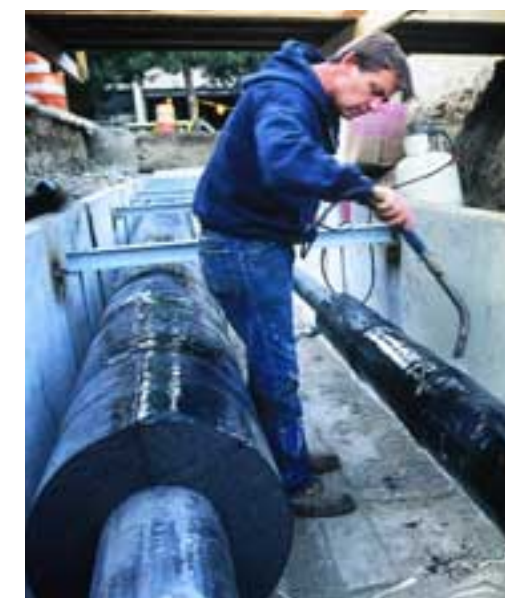
StrataFab® sections were installed in succession and butted against one another with PITTWRAP® butt stripes at the interfaces, and heat sealed.
